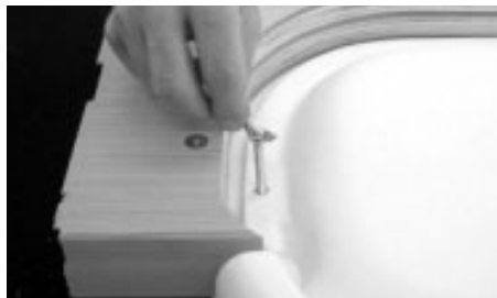
2 - Tighten the wing nut on the threaded bar until it touches the washbasin (see photo 3).
