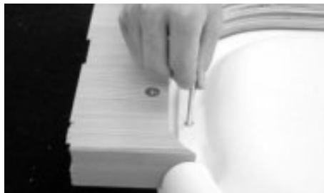
1 - Tighten the threaded bar on the bush on the washbasin.
