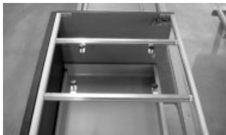
Adjust the pins until the washbasin is resting on it.
